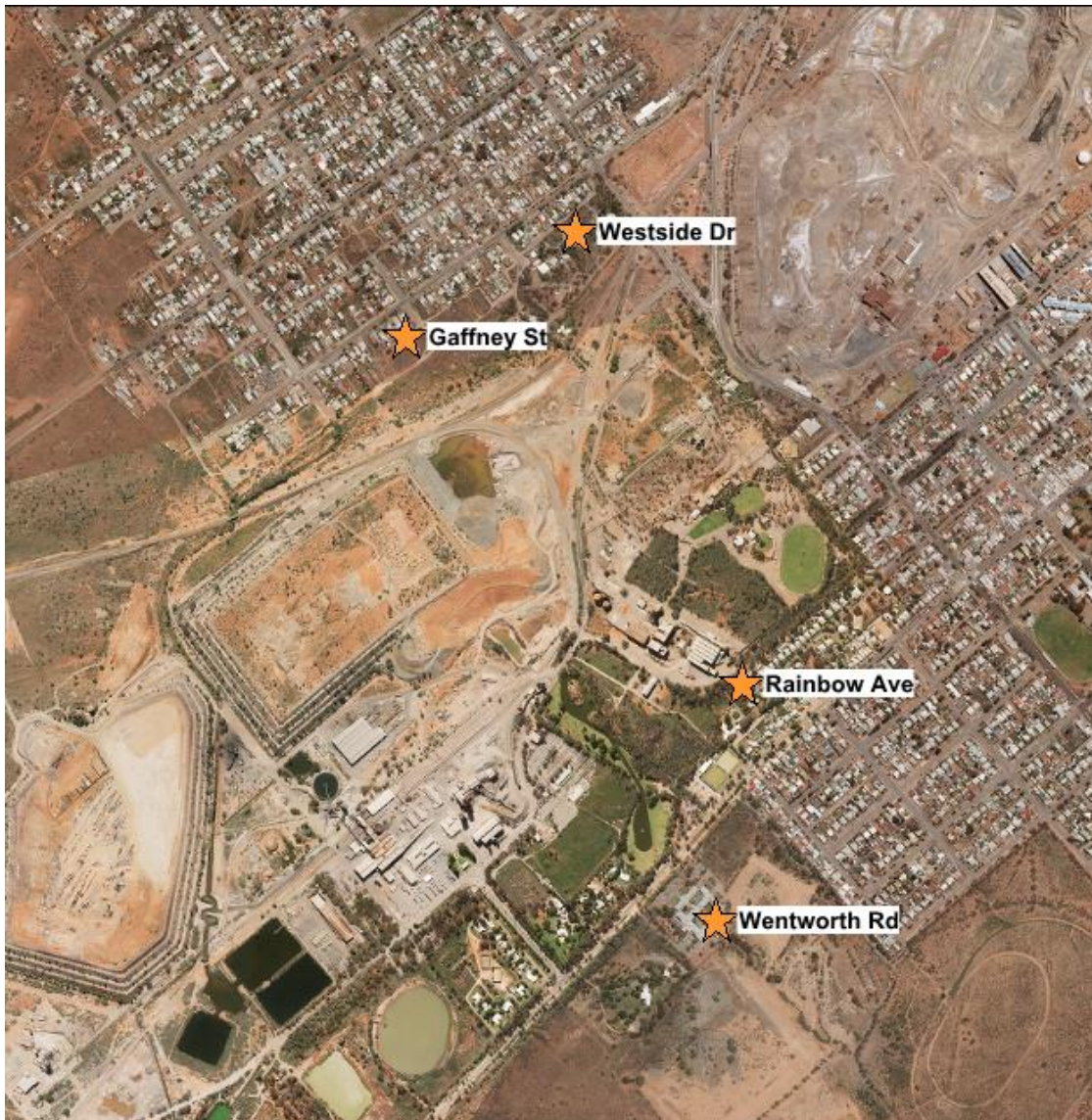
Figure 6. Location of EPL2688 blast monitors.
